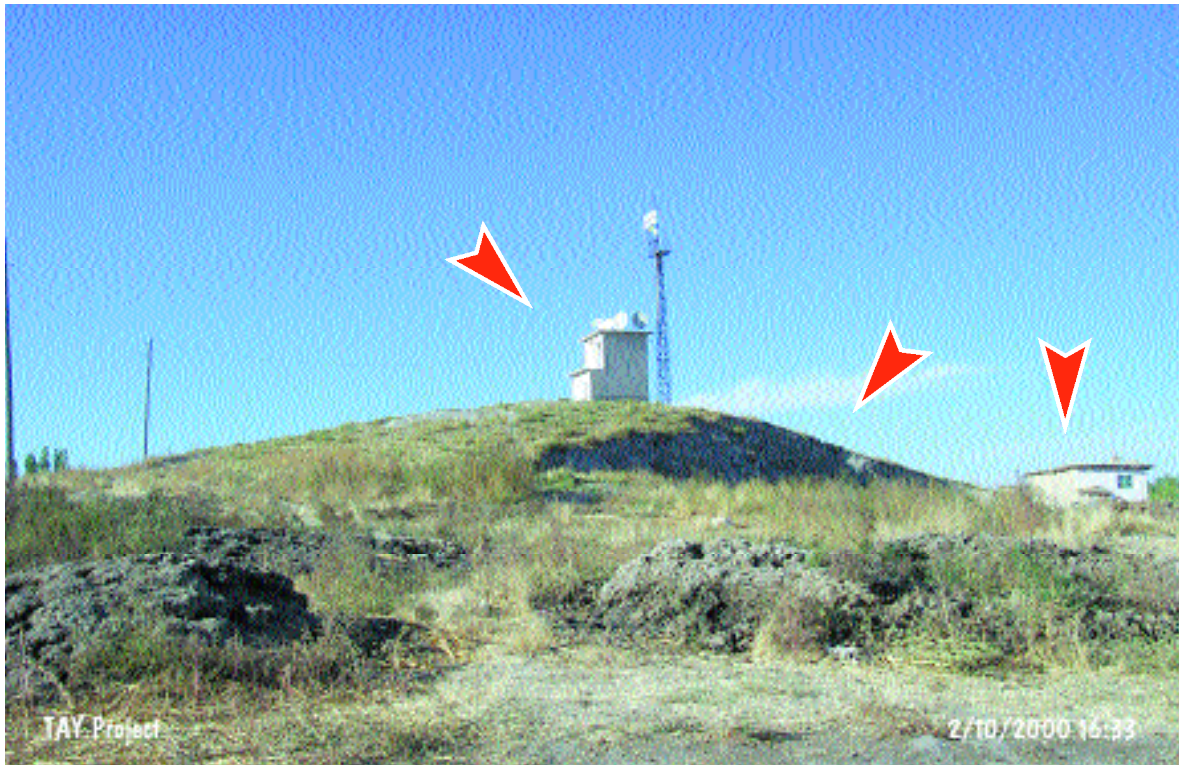
Çobanlar Kadıyük (mound): EBA. A broadcasting station, a TV/radio transmitter, power towers on the top and a house on the southern slope. The eastern sector cut away by the municipality.
